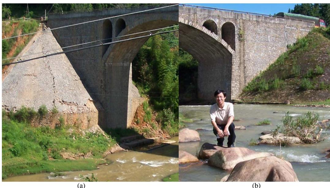
**Fig. 5** (a) In a section of a tributary of the East River without ribbing structures the channel bed is eroded down by about 2 m and the bridge is endangered by the incision; (b) In another section of the same stream with ribbing structures the channel bed remains stable.
